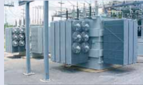
VEC completed a major upgrade of the Lantana substation in Cumberland County in June.
