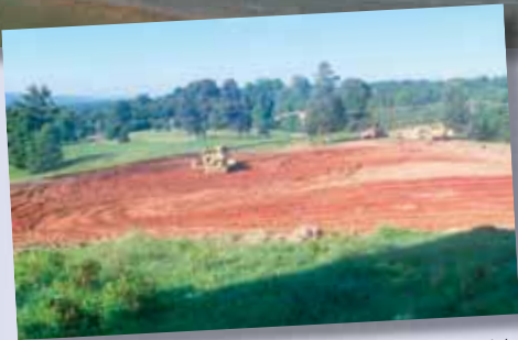
Work is progressing on VEC's new Georgetown substation which is scheduled for completion in the fall of 2014.
