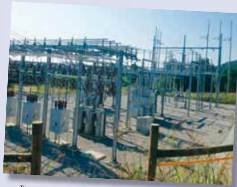
The newly completed Byrdstown substation in Pickett County was energized on September 14, 2012.
