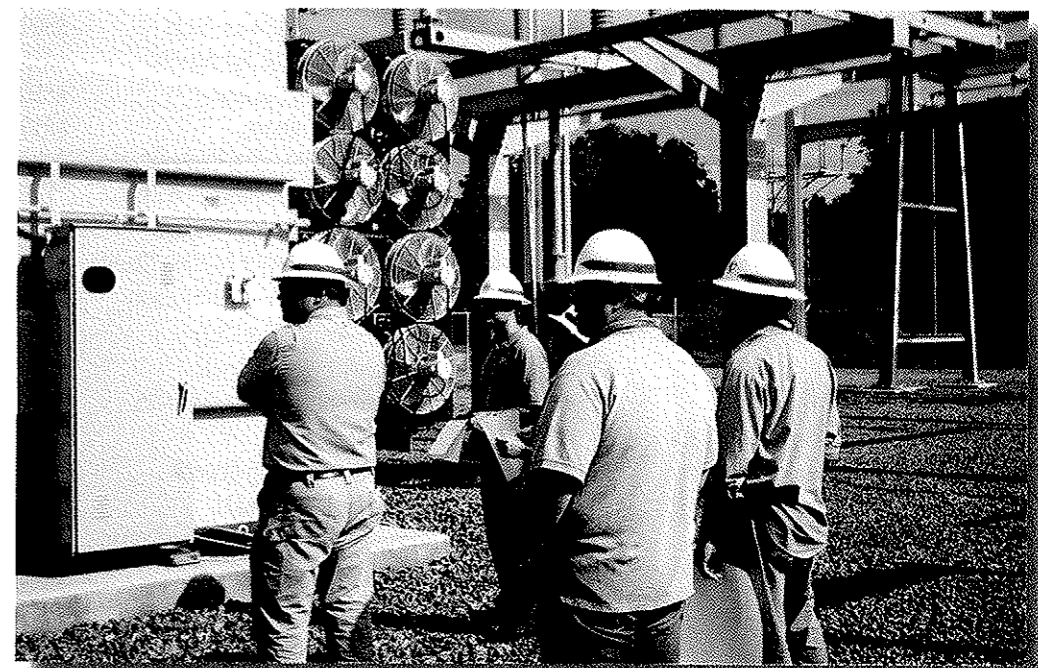
VEC engineer Matthew Teague trains dispatchers and linemen on manual and remote operation of VEC's new Georgetown Substation.
