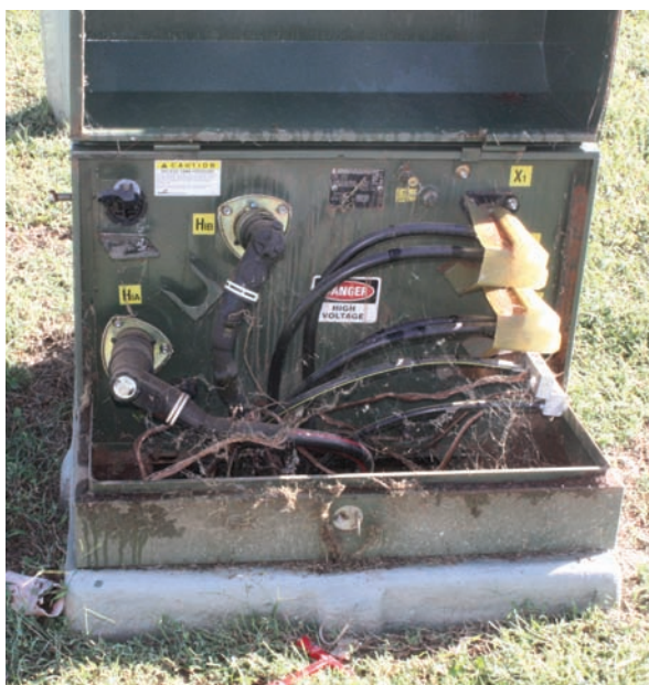
Single Phase Pad Mount Transformer Open
