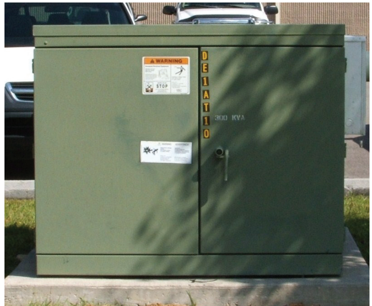
Three Phase Pad Mount Transformer
