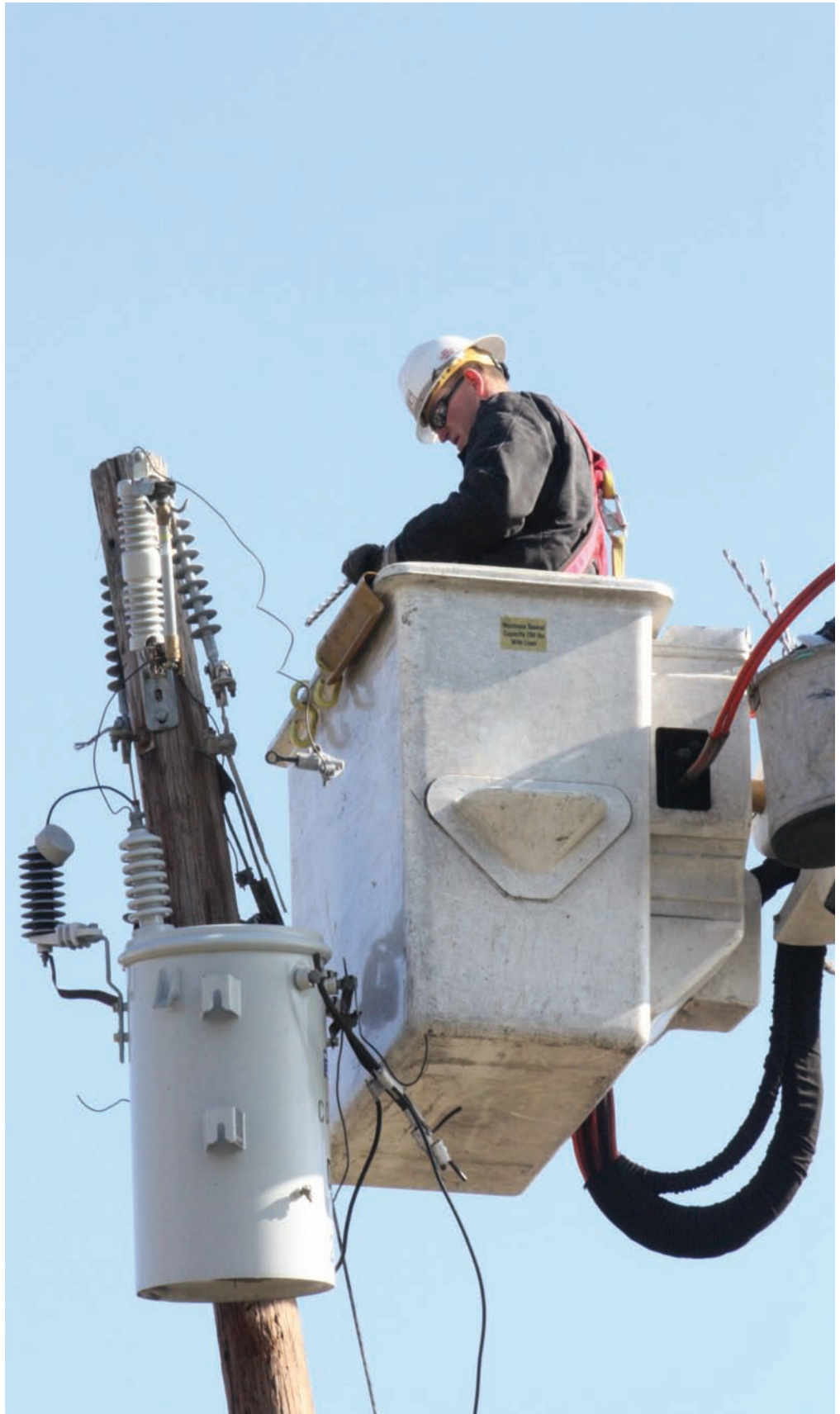
The Pole Mounted (overhead) Transformer resembles a large can.
