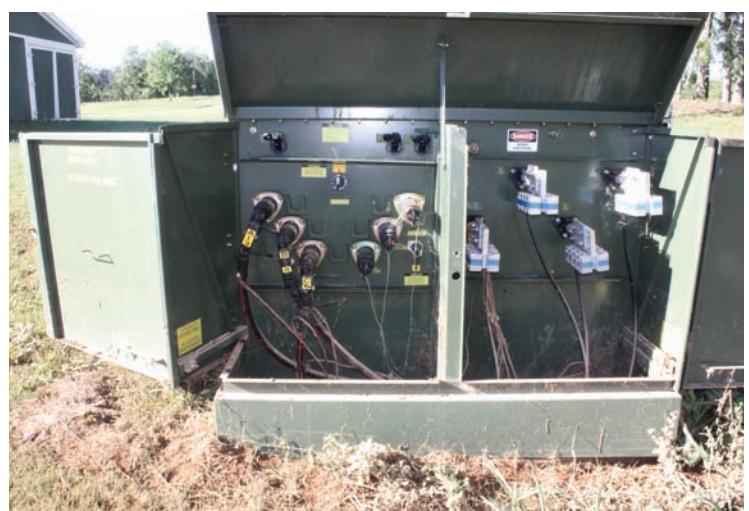
Three Phase Pad Mount Transformer Open
