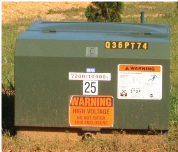
Single Phase Pad Mount Transformer
