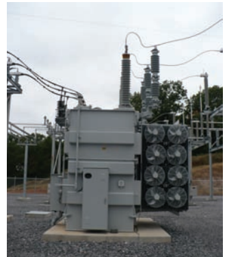
Substation Transformer
