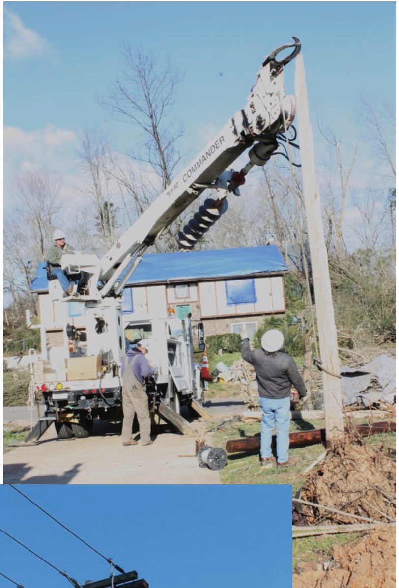
Digger-Derrick Truck Pole Setting
