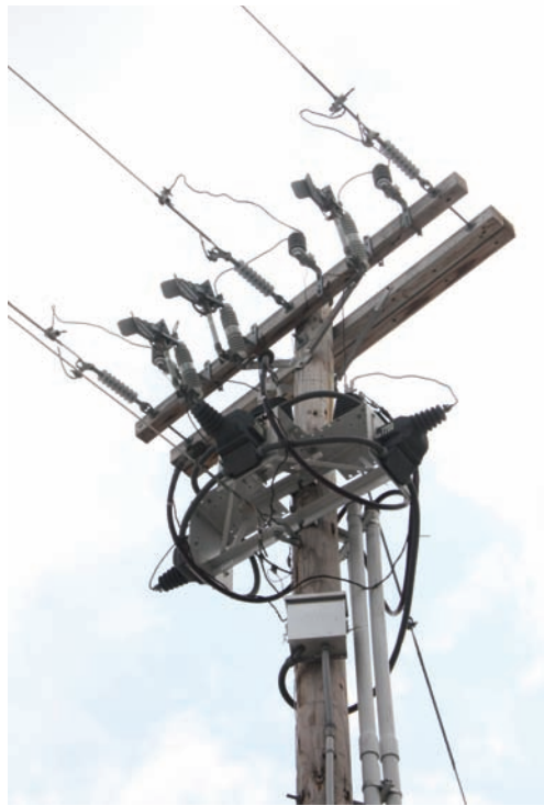
Primary Metering Detail
