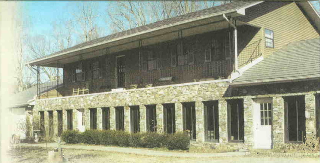
A front view of the Pursley home shows the attractive solarium that helps reduce energy bills.
