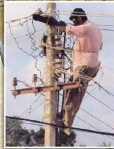
*Working mainly with a pair of needle-nose pliers, and without benefit of safety equipment other than a rope to tie himself to the pole, this electrician in Burma Nagar, India works to restore power.*
