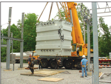
Contractors from Southwest Electric and Volunteer Energy Cooperative employees move the 75 ton transformer into place at the Sugar Grove Substation in lower Bradley County
