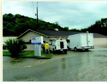
VEC's Spring City Customer Service Center suffered from severe flooding again in 2004.
