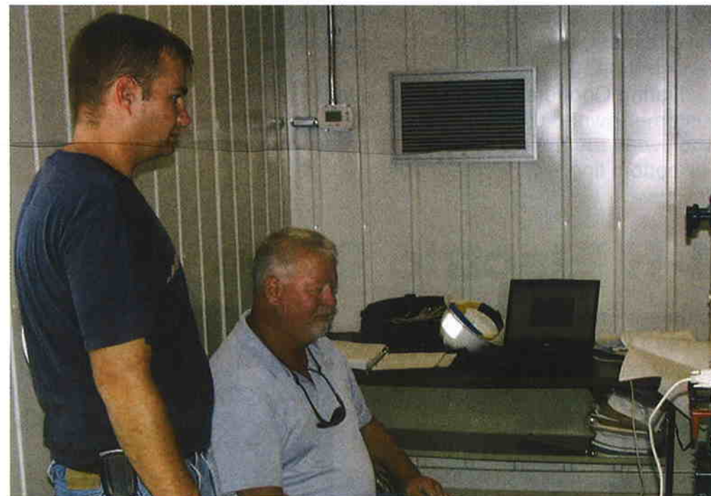
Matthew Teague and Darrel Crisp monitor progress as VEC energizes the new South Bradley Substation. The new substation was put into operation on July 17.
