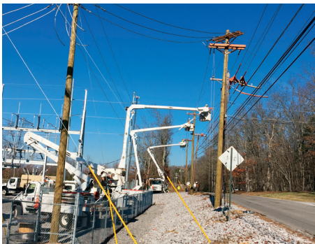
Crews work to energize the new West Fairfield Substations.
