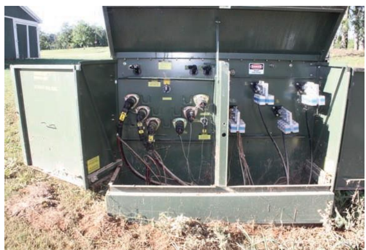
Three Phase Pad Mount Transformer Open
