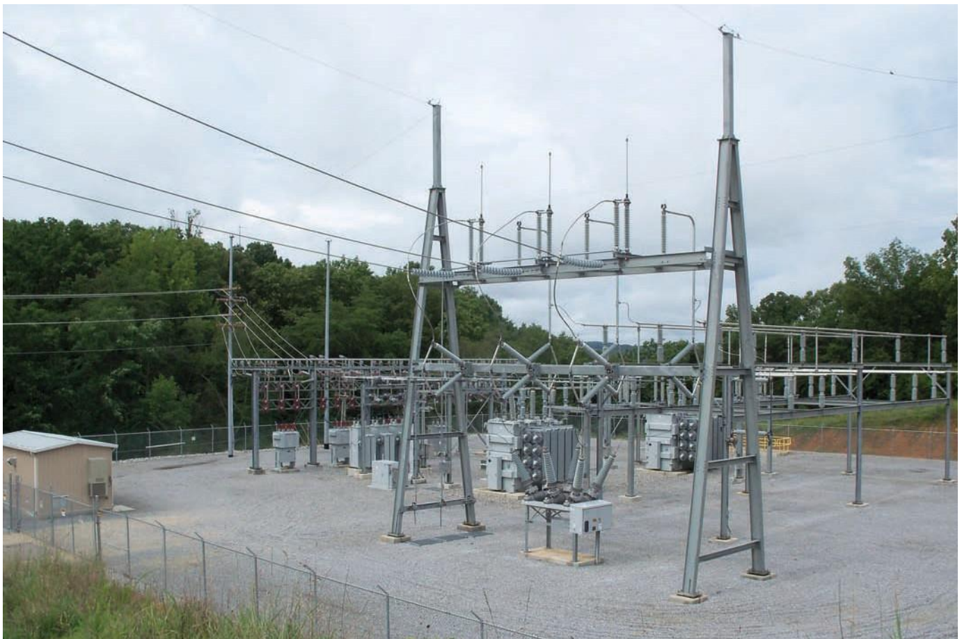
Hiwassee Substation - Bradley County
