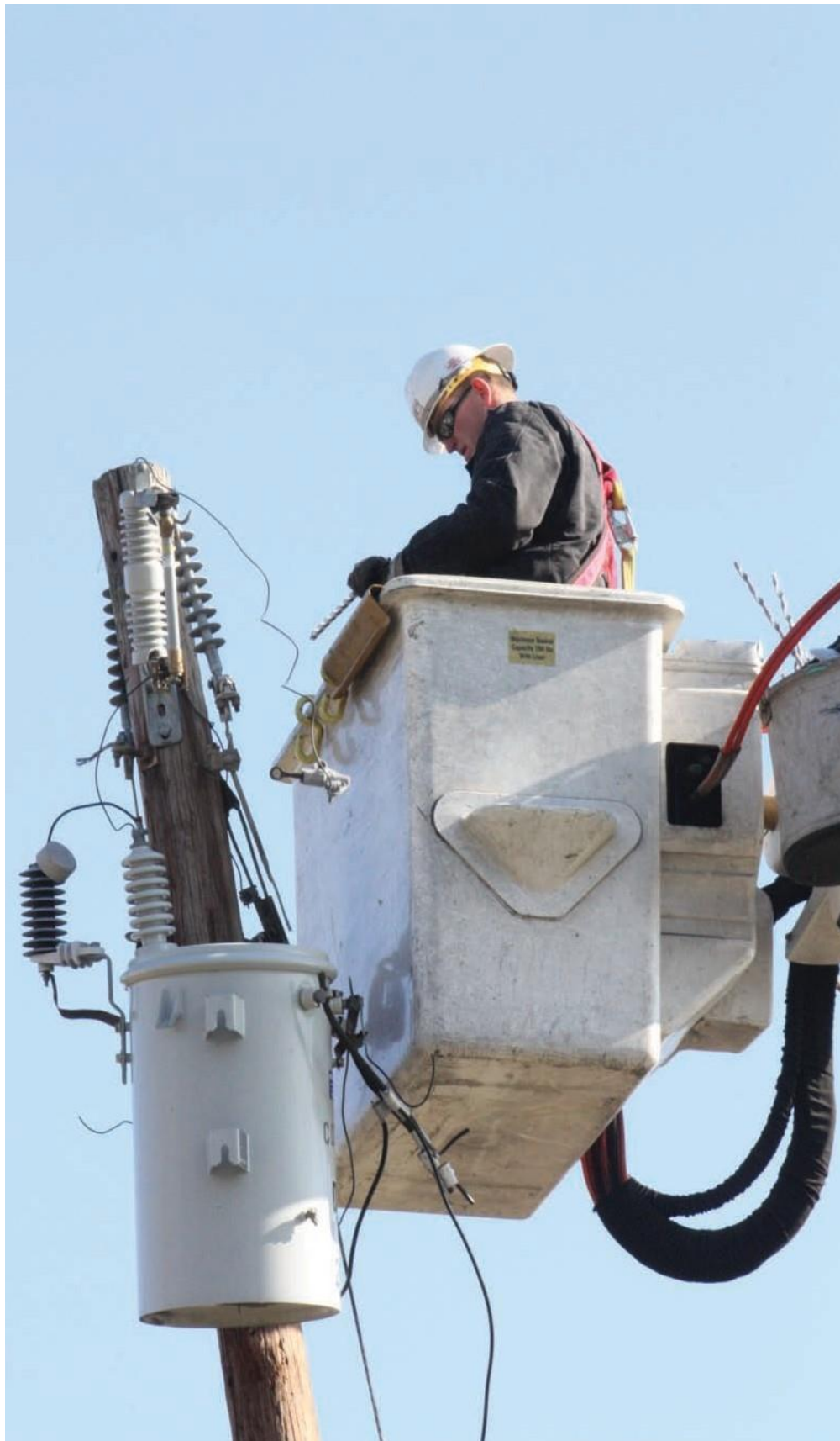
The Pole Mounted (overhead) Transformer resembles a large can.
