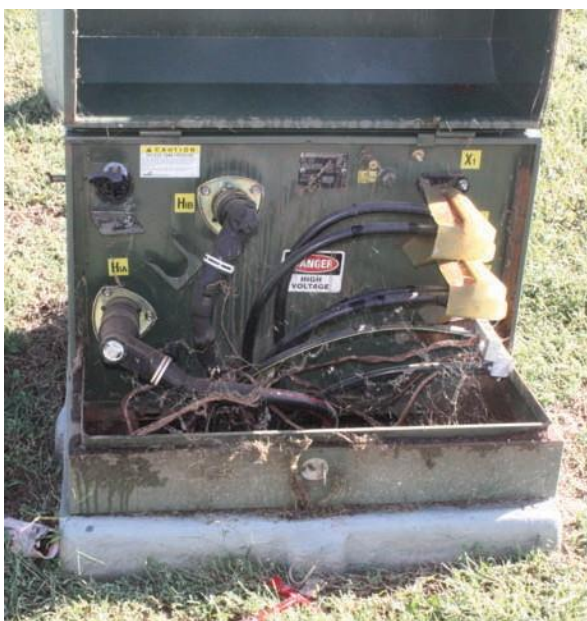
Single Phase Pad Mount Transformer Open
