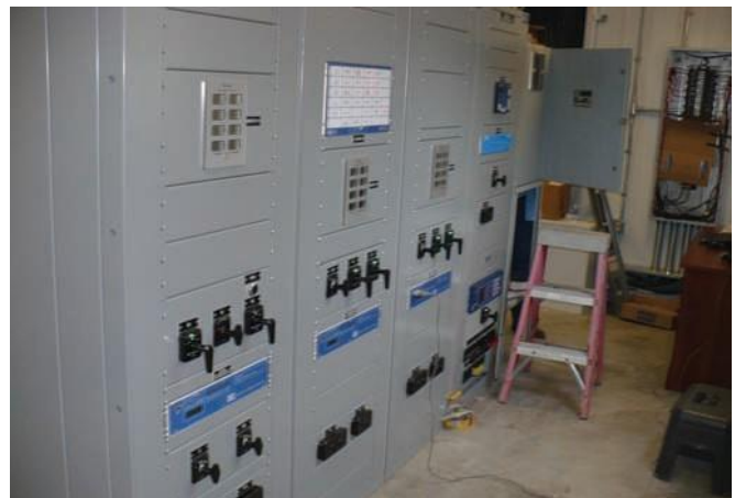
Substation Control Panel
