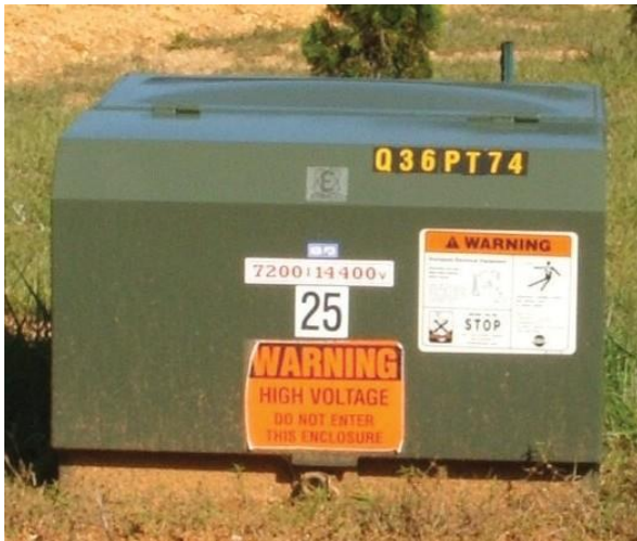
Single Phase Pad Mount Transformer
