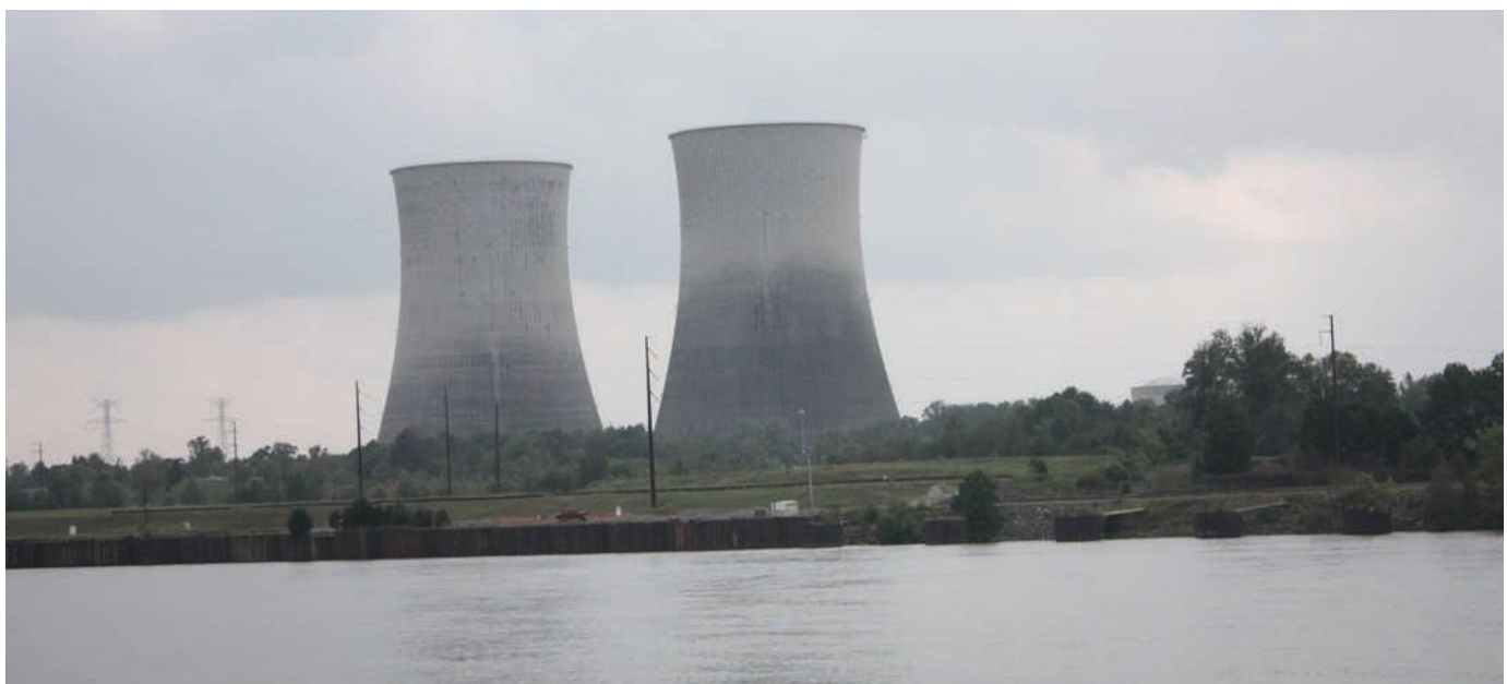
TVA Nuclear Cooling Towers
