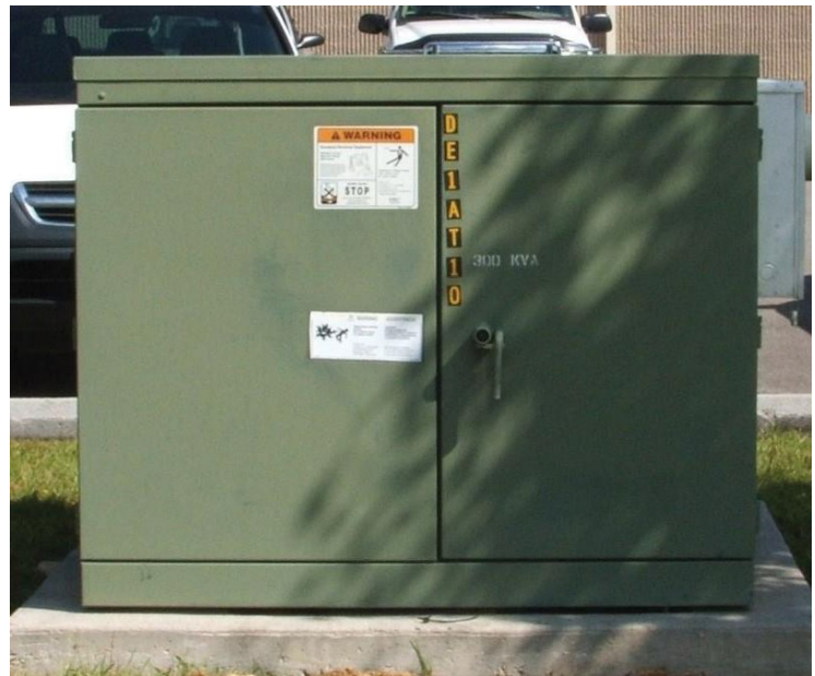
Three Phase Pad Mount Transformer
