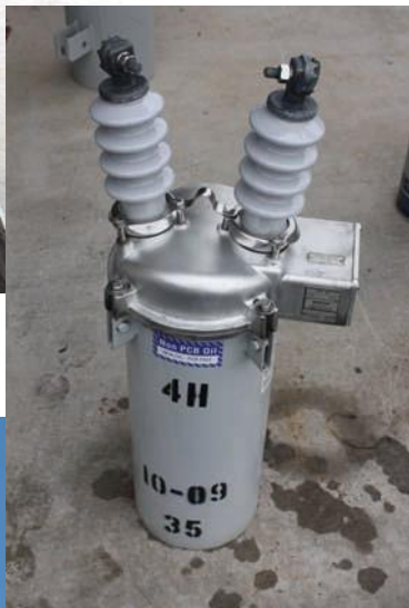
Single Phase 35 amp Recloser
