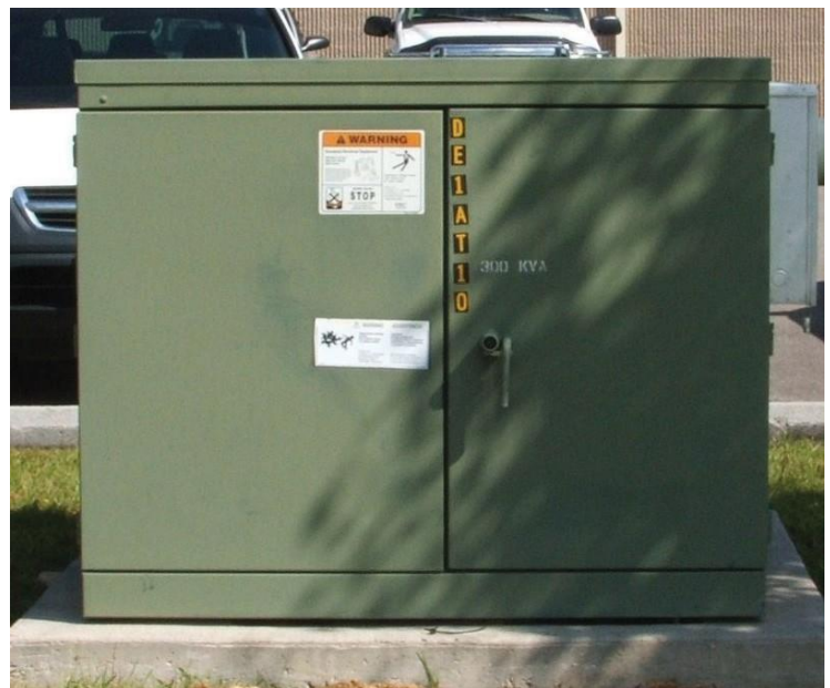
Three Phase Pad Mount Transformer
