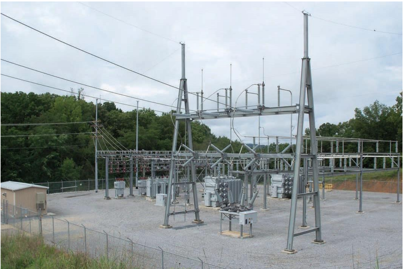
Hiwassee Substation - Bradley County
