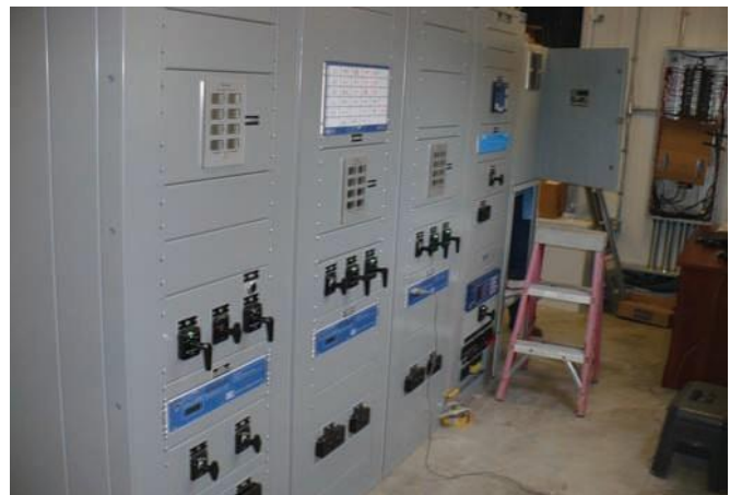
Substation Control Panel
