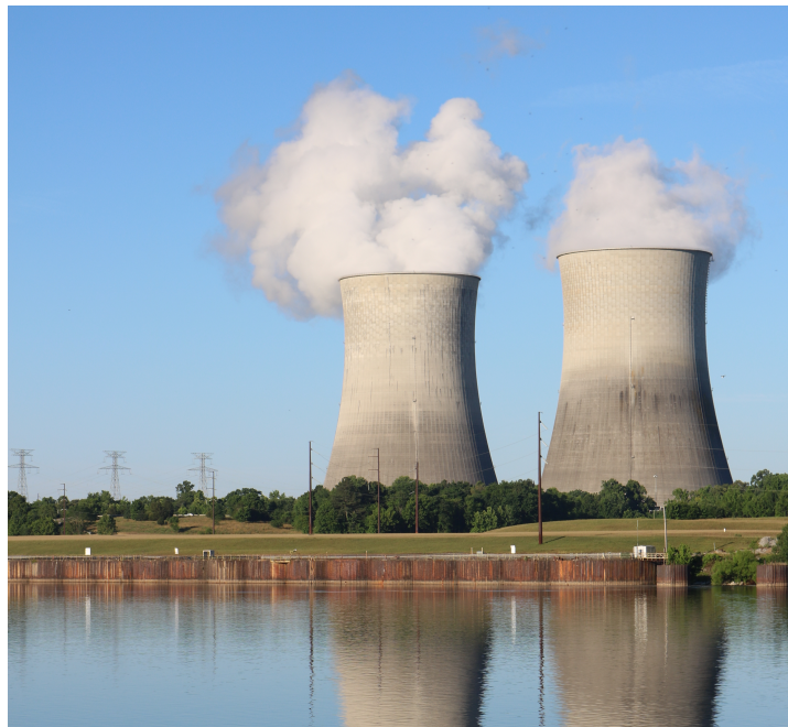
TVA Nuclear Cooling Towers
