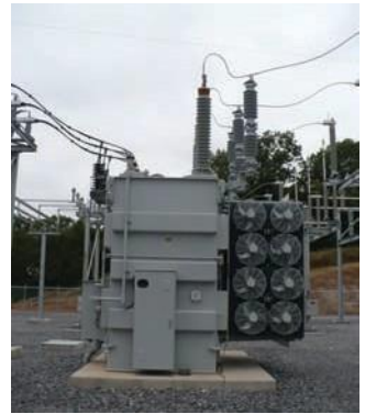
Substation Transformer
