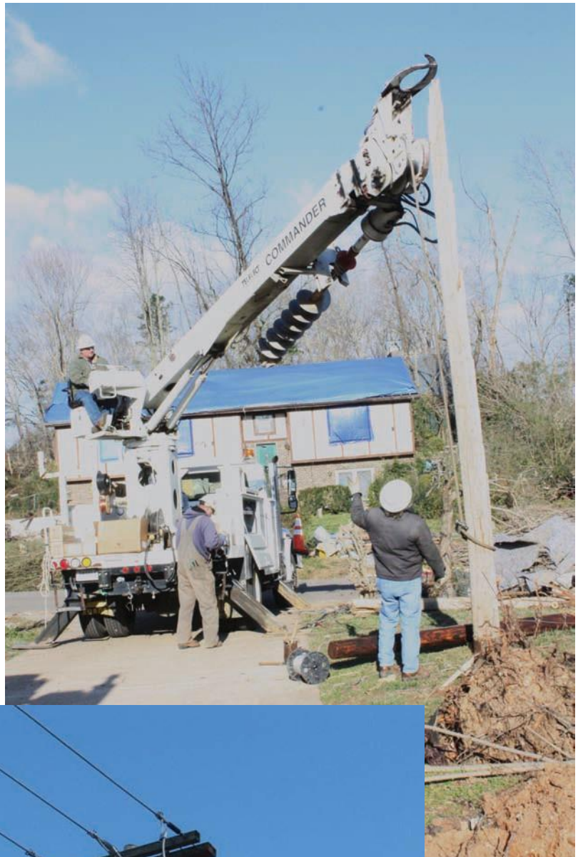
Digger-Derrick Truck Pole Setting
