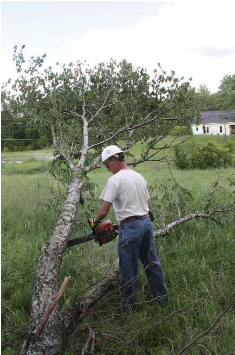
Clearing Rights-of-Way to Protect the Distribution System is a Non-Stop Job.
