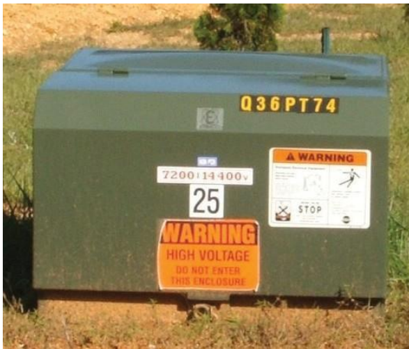
Single Phase Pad Mount Transformer
