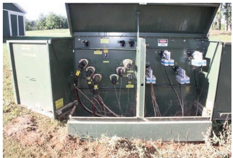
Three Phase Pad Mount Transformer Open
