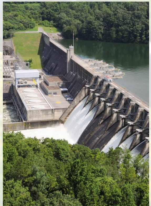
TVA utilizes water as an energy source at its dams.
