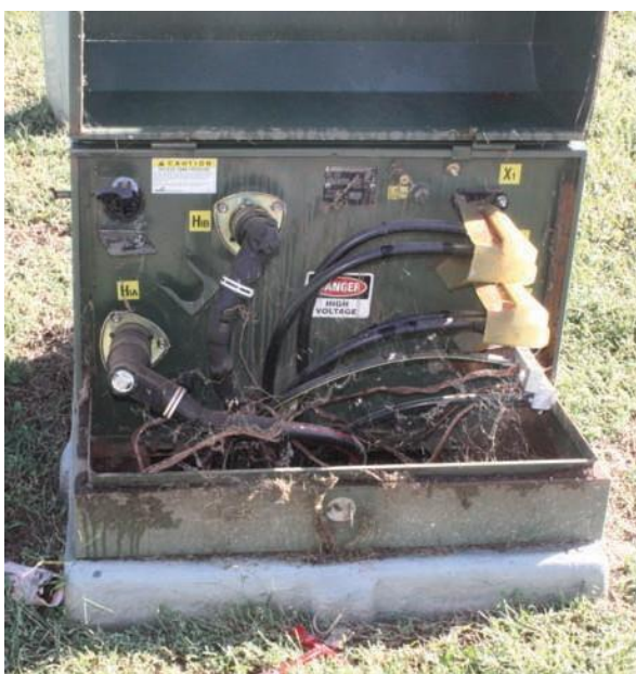
Single Phase Pad Mount Transformer Open
